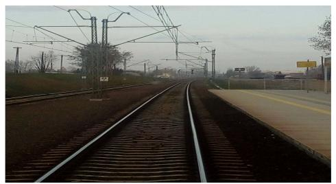
Fig. 3. Support structures blocking the train driver's view of the trail
