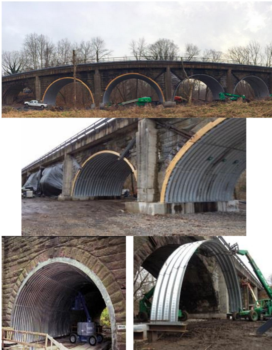
3. Strengthening the stone vaults of brick railway bridge [5]
