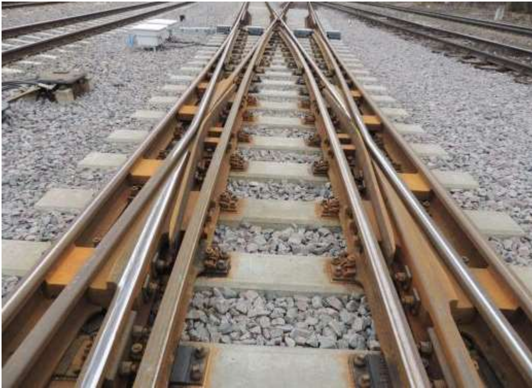
6. View group of ordinary crossings and double-steering crossover Rkpd 60E1-190-1 :9 by KZN "Biezanow" (pic. KZN "Biezanow")
