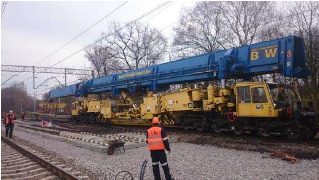
2. Installation the steering of crossover Rkpd using a crane Gottwald GS150.14.TR
