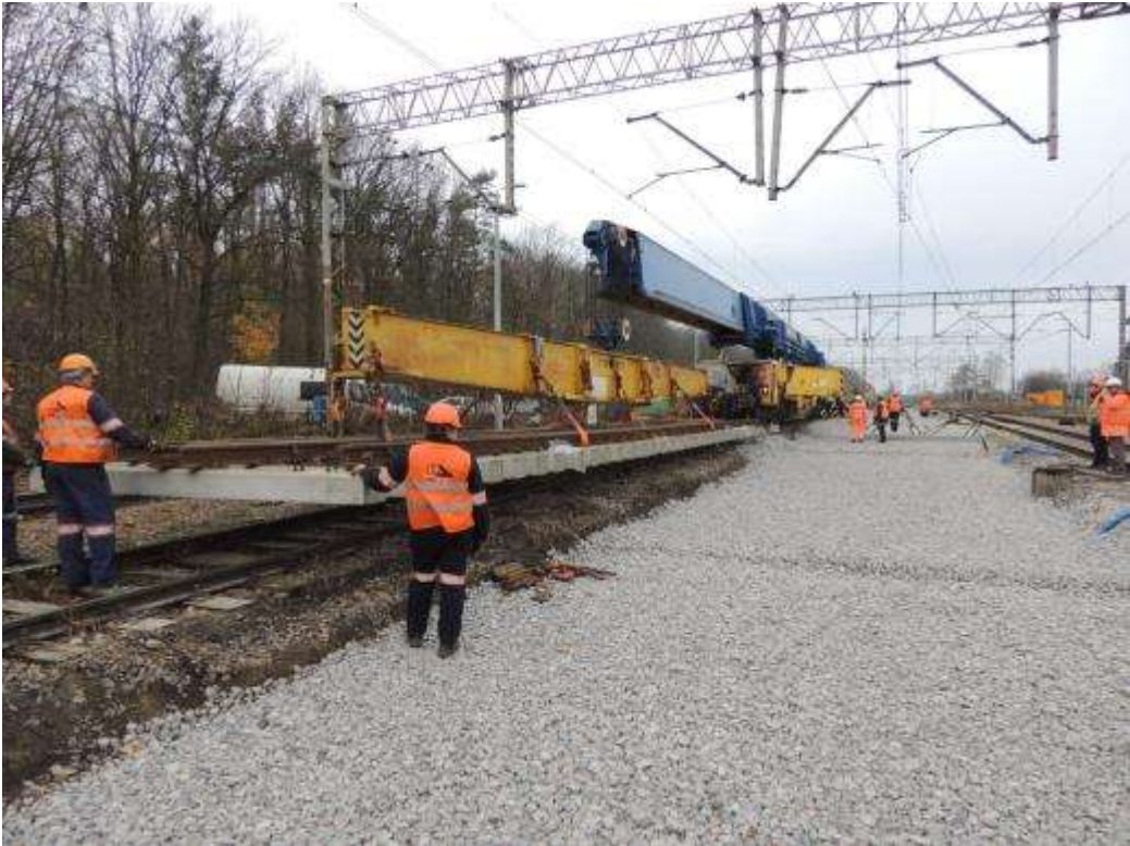
3. Installation of crossover switch Rkpd using crane Gottwald GS150.14.TR
