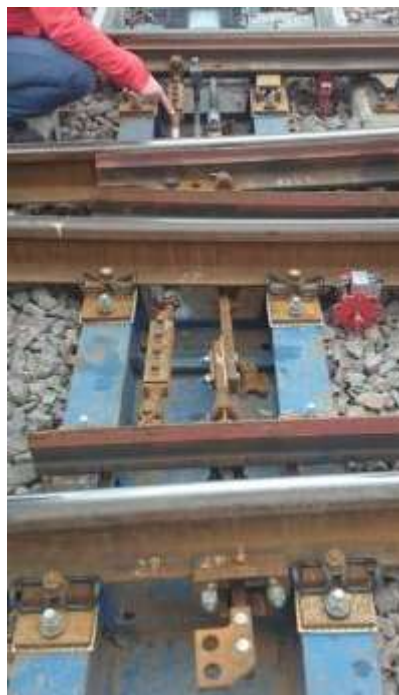
10. complex bearer with the closure of adjusting in the switch of Track Tec KolTram Sp. z o.o.
