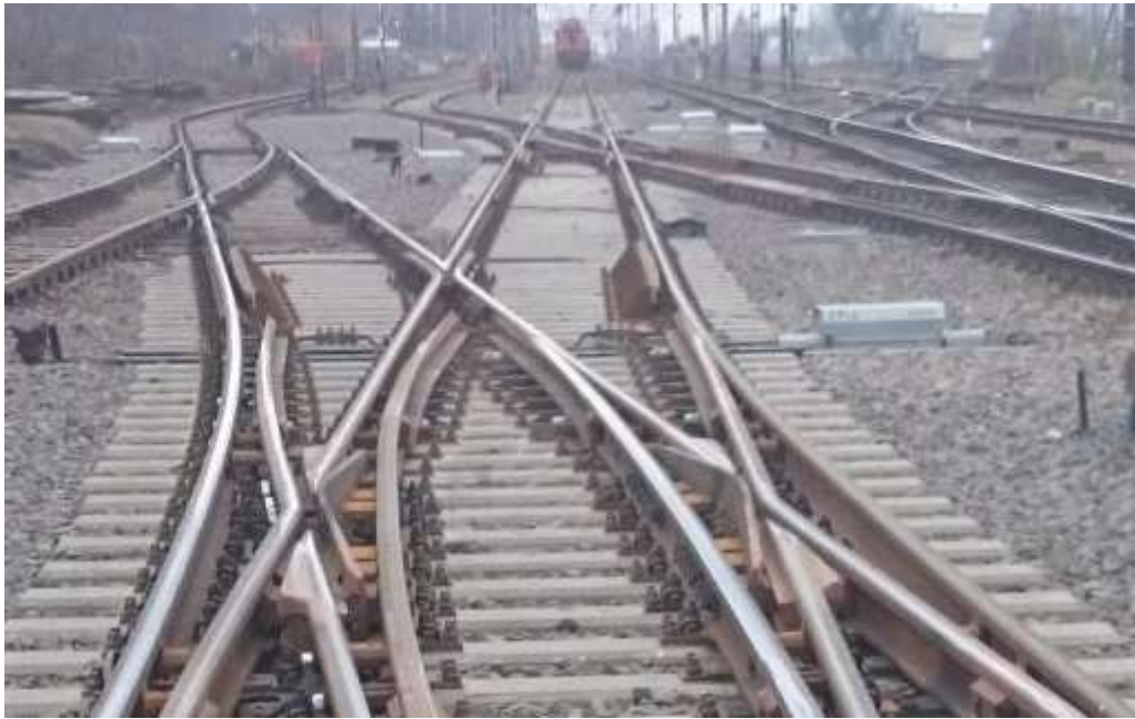
9. View group of double crossings and steering switch of Track Tec KolTram Sp. z o.o.
