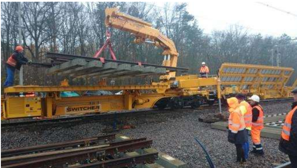
5. Building over element ordinary frog with a crane platform of "Switcher"
