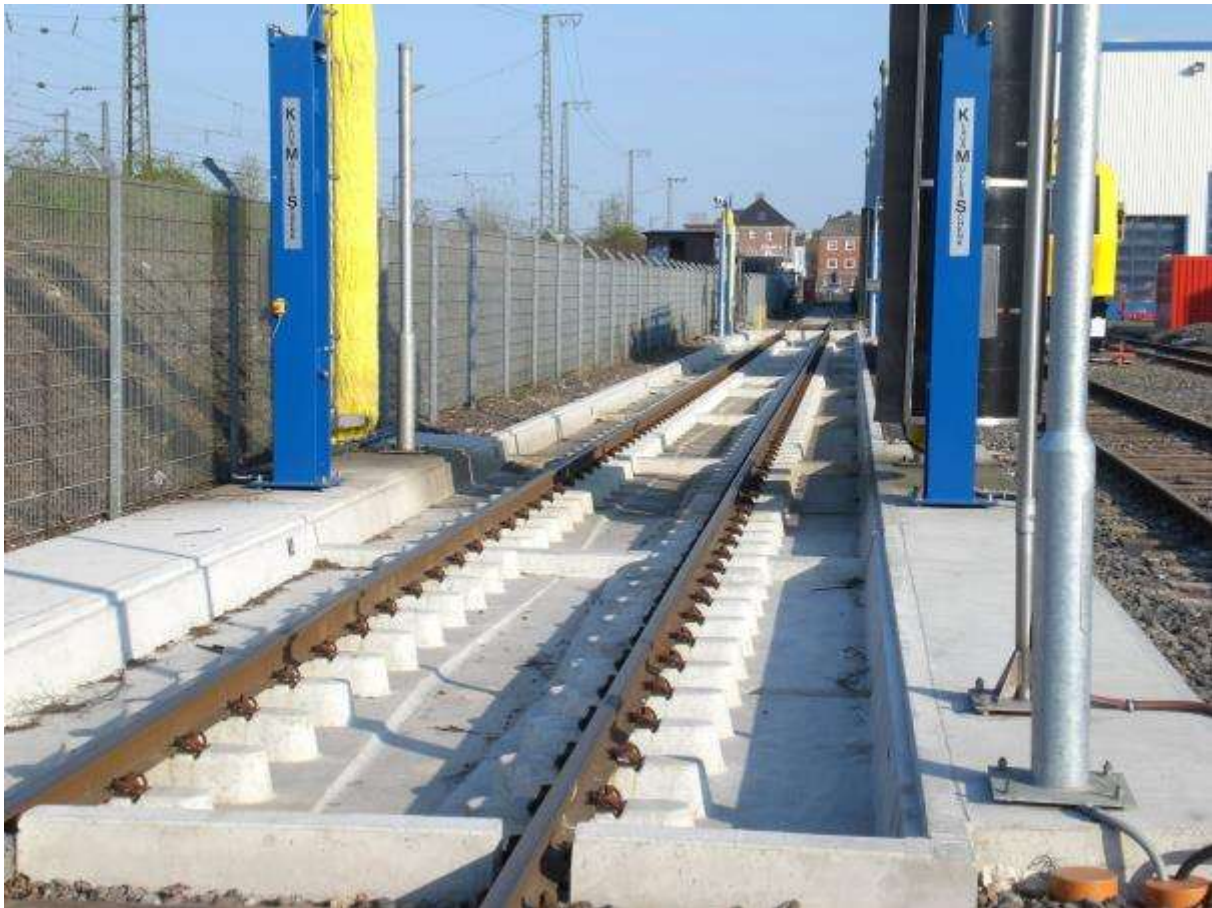
2. Ecological point of vehicle washing stations, made on sealed track tubs GTW system (Pic. BFL Lauchhammer)
