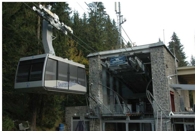
4. 60 passenger cabin on the section I - lower station Kuznice.
