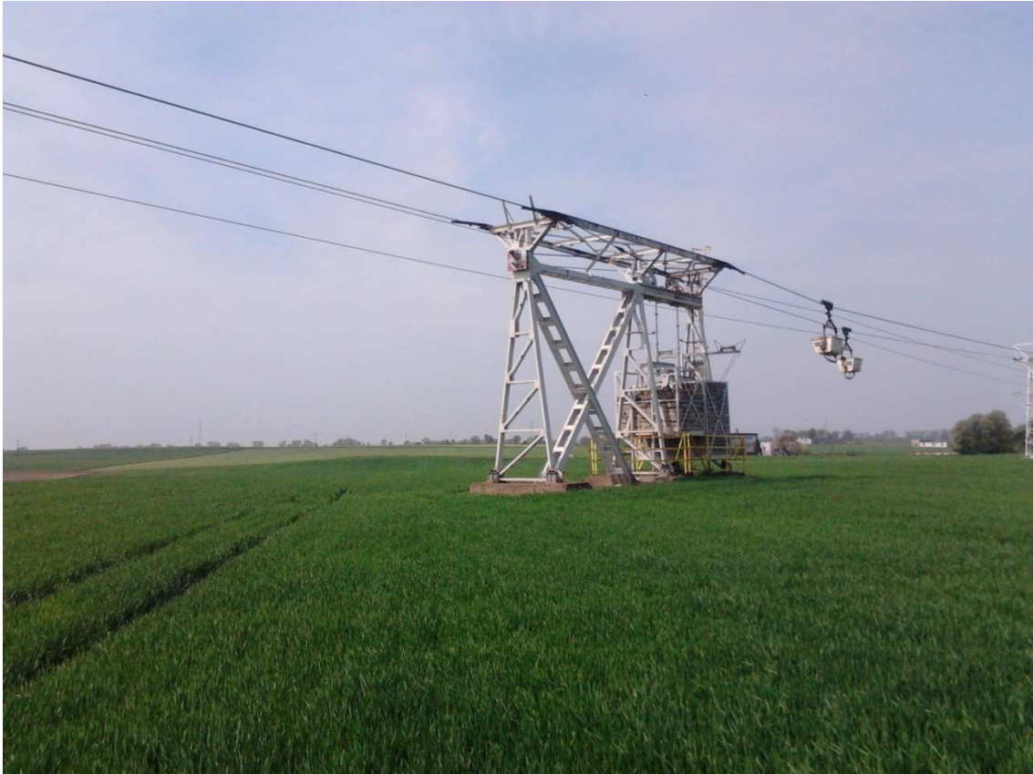
8. Station tensioning ropes carrying adjacent ropeway sections.
