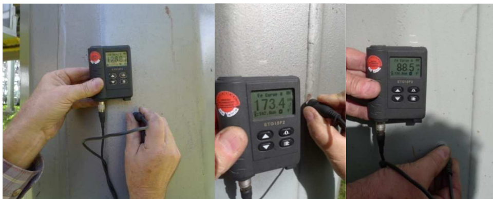
13. Sample pole measurements of the support: a) native material, b) weld c) SWC + magnetized area MT.
