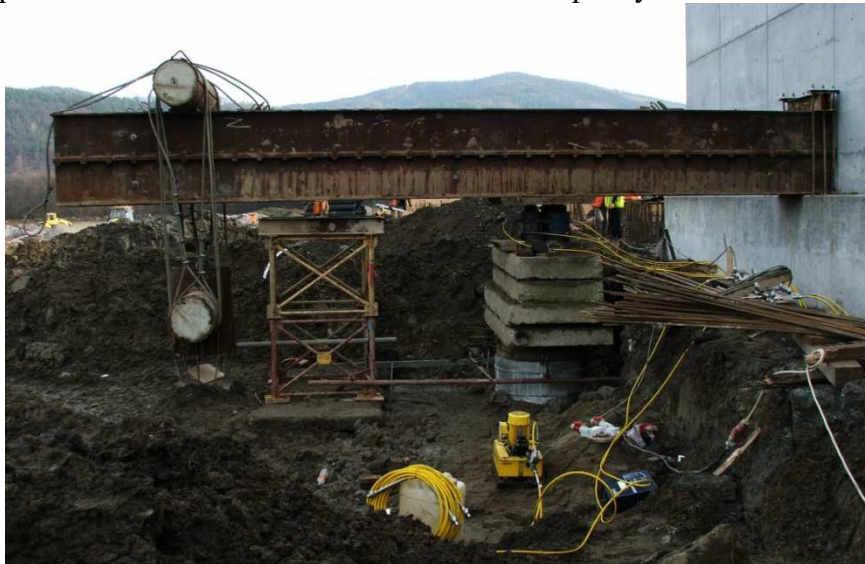
3. Emplacement for the test load stone column
