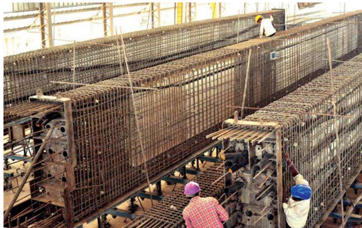
3. Preparation of reinforcement [12]
