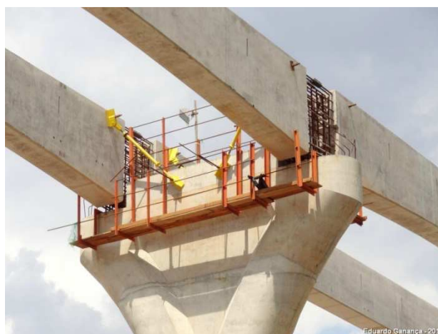
9. Stabilization of girders after assembly on a support [8]
