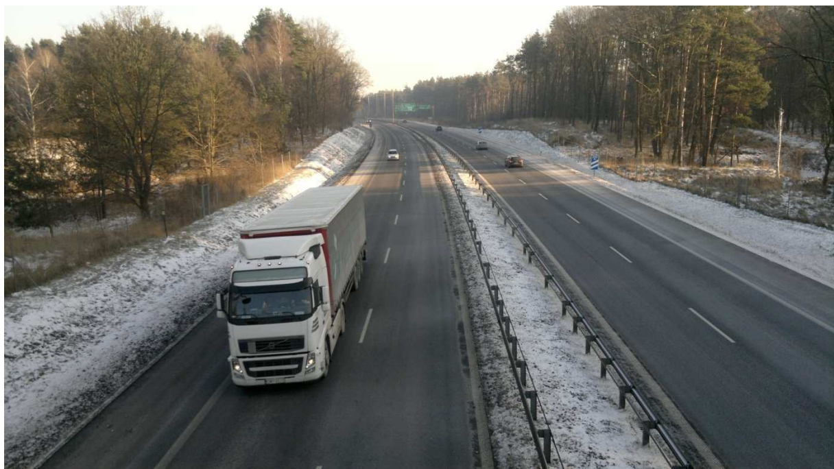
3. Section of the A6 motorway near the road junctions of Szczecin Kijewo (starting point) Source: own elaboration
