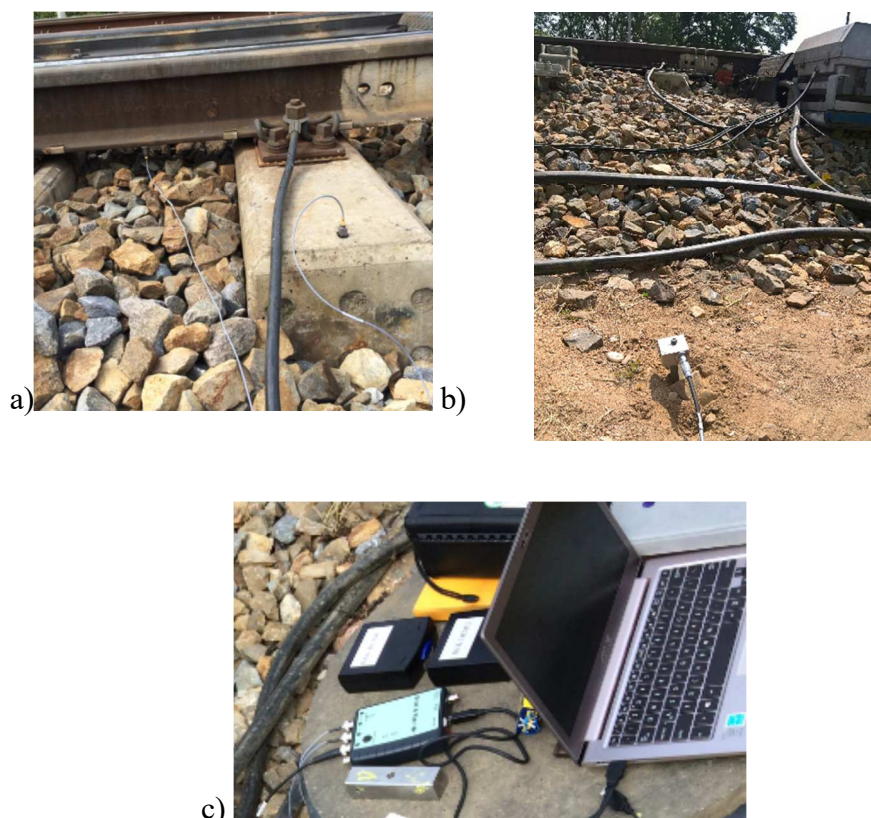
9. Measuring apparatus and location of measurement sensors in the turnout, a- sensors on the rail and sleepers, b- sensor in the substructure, c-measuring apparatus, Siedlce August 2016
