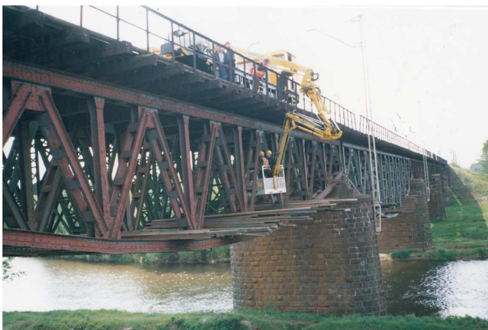
2. Detailed review of truss girders of the bridge spans
