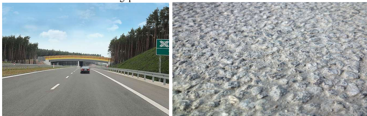
4. The S8 expressway - "discovered aggregate" technology
