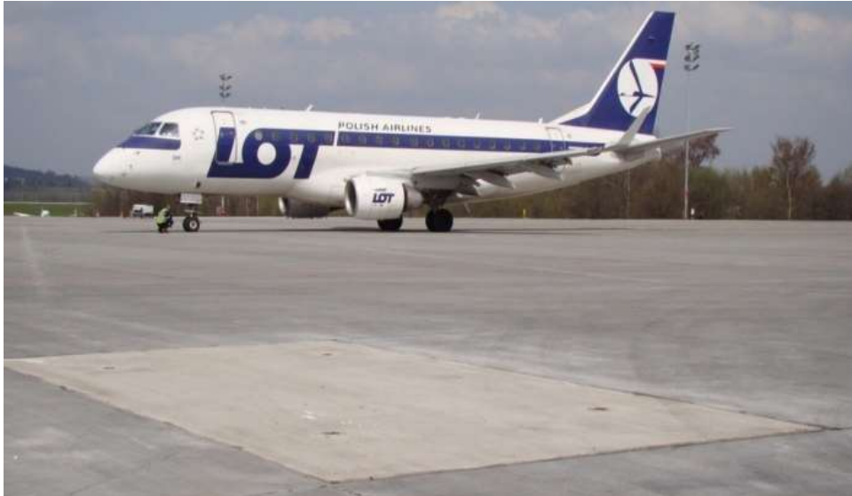
4. Prefabricated slab on the apron's airfield pavement at Kraków-Balice airport
