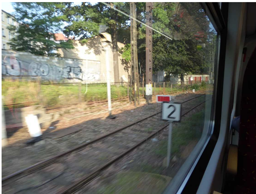
23. Signal D 1 "Stop" given by the stopping disc on the 283 line on the western exit head of the station in Jelenia Góra seen from the train on the 311 line
