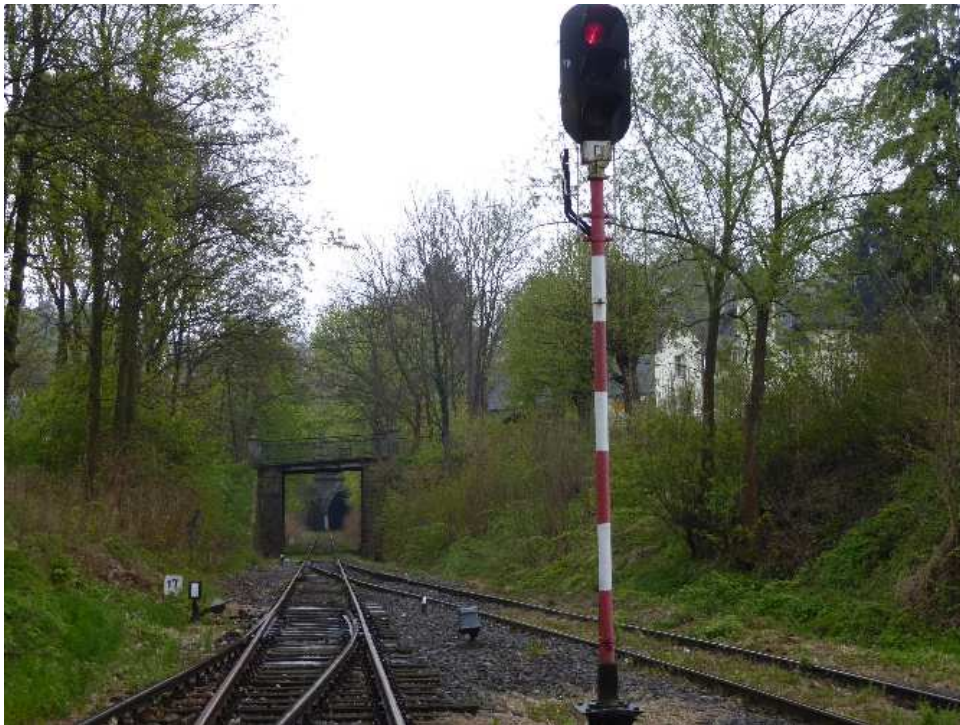
17. Road bridge and tunnel visible from the Wleń station
