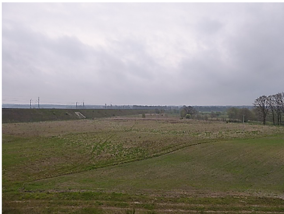
5. View of the embankment and viaduct over the Kwisa river, on the E30 railway line from line 283 near Zebrzydowa
