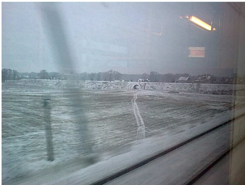
4. View of embankment line 283 above the viaduct on the Kwisa River near Zebrzydowa on the E30 line
