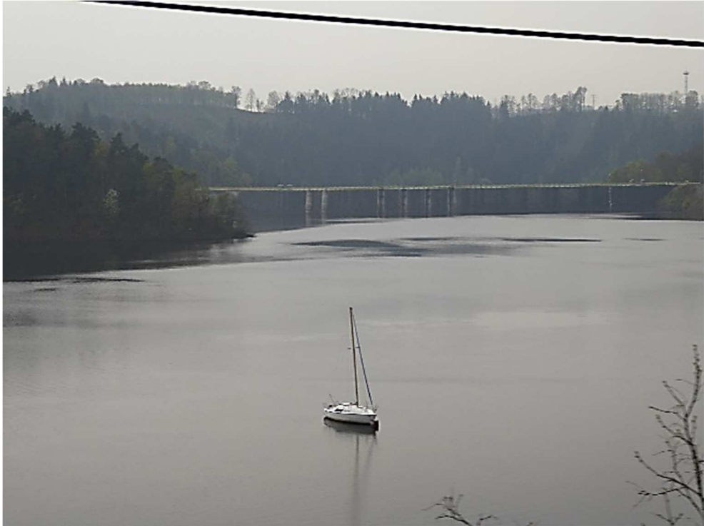
19. Pilchowickie lake and cable
