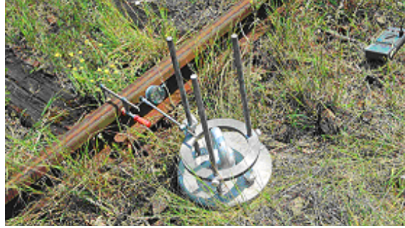
9. Measurement of the longitudinal displacement of a railway track depending on temperature (author's photo)
