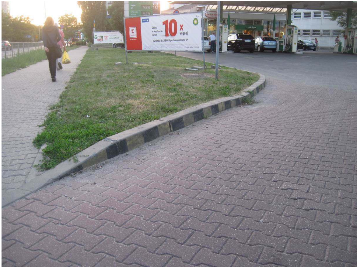
2. Example of contrasting curb painting improving its visibility - Warsaw/Poland
