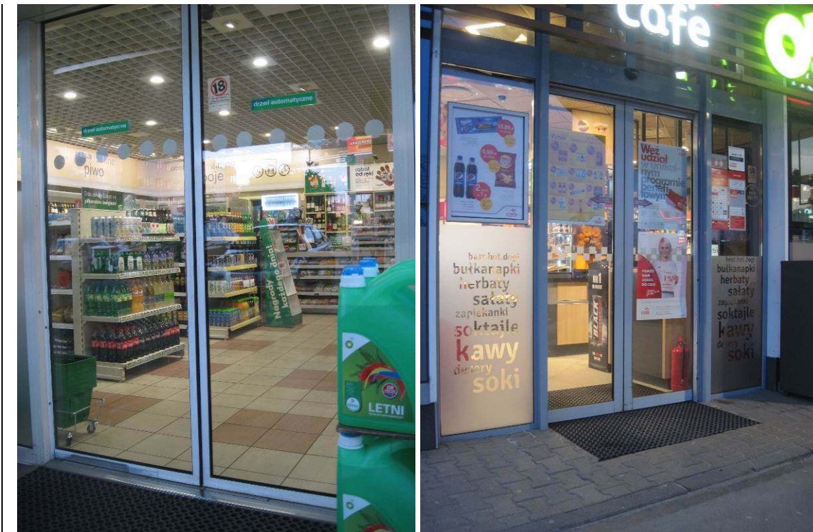
6. Glass door with information indicating glazing and advertisements enhancing this information - Warsaw/Poland.
