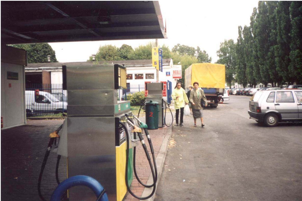
11. The construction of the station without a pavement caused dangerous pedestrian traffic through the station area - Poland
