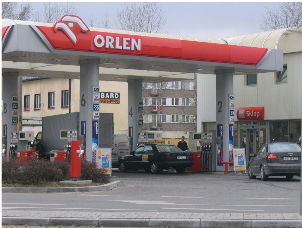
3. Roofing of the refueling zone and access to the building has a positive effect on the safety and comfort of movement of accelerated drivers and passengers - Siedlce/Poland
