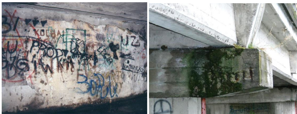
14. Neutral inorganic pollutants (left) and organic surface pollutants in the form of algae (right)
