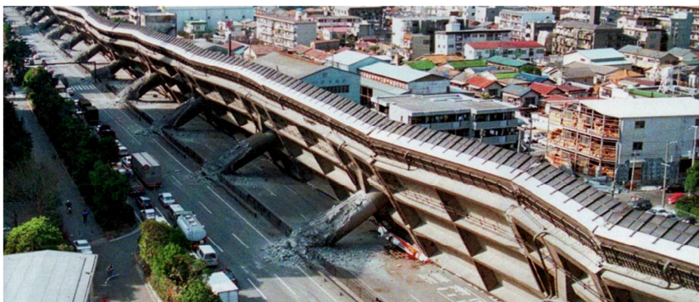
15. Changing the position (rotation) of the entire bridge structure as a result of an earthquake, combined with deformations as well as losses and loss of material continuity
