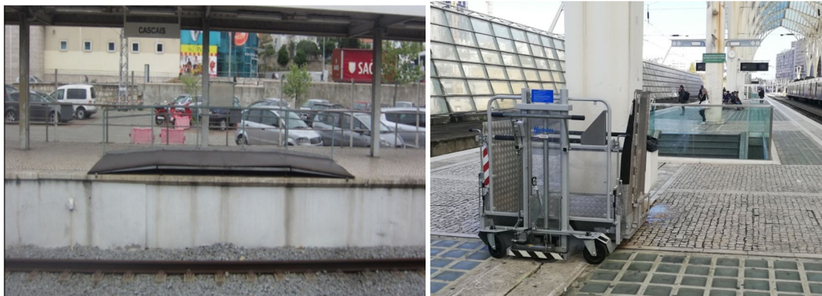
4. Raising part of the platform (a) and a portable platform lift (b)
