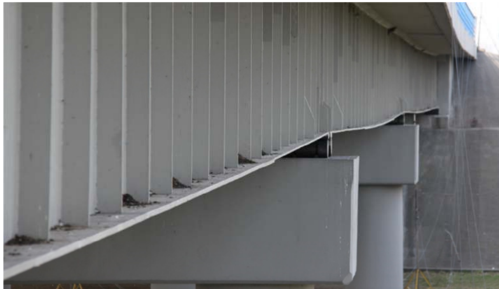
2. Permanent deflection of the main spans
