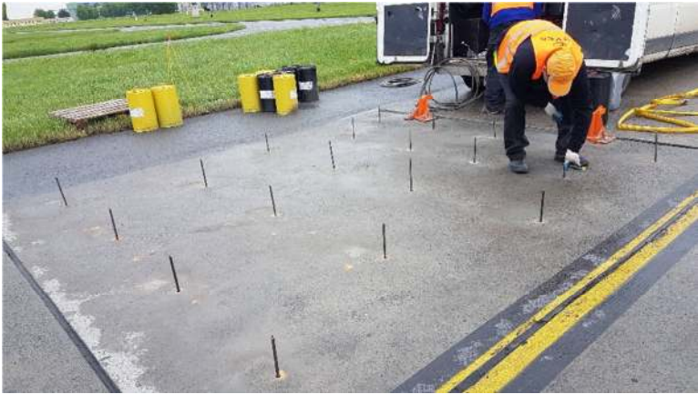
7. Embedding in drilled holes, steel injection lances
