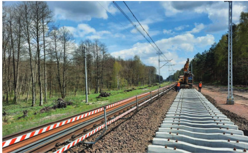
1. Railway safety barriers
