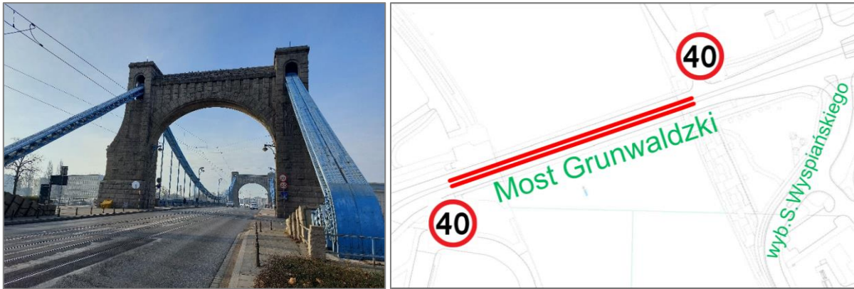
1. Grunwaldzki Bridge, view from Grunwaldzki Square
