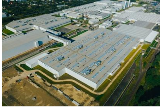
14. The new Opel factory from a bird's eye view [5]
