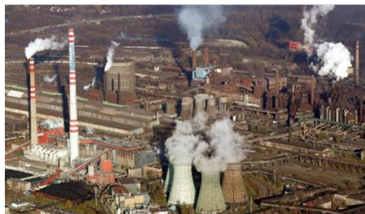
15. ArcelorMittal's metallurgical complex in Ostrava [14]
