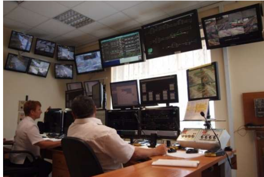
5. Equipping LCS Drzewica with modern solutions for managing railway traffic.
