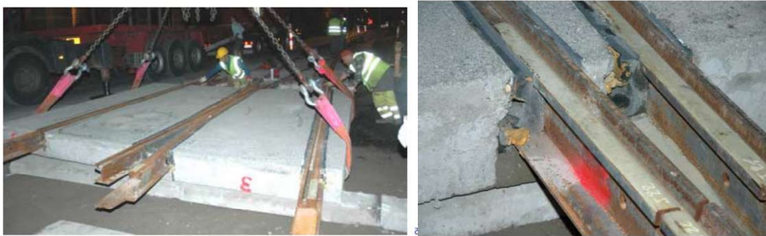
2. Installation and assembly of a turnout in a prefabricated slab – Brussels [5]
