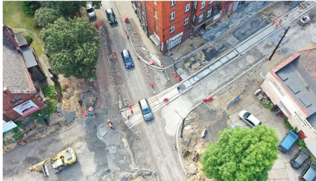
3. Prototype installation of a turnout in prefabricated slabs in Bytom
