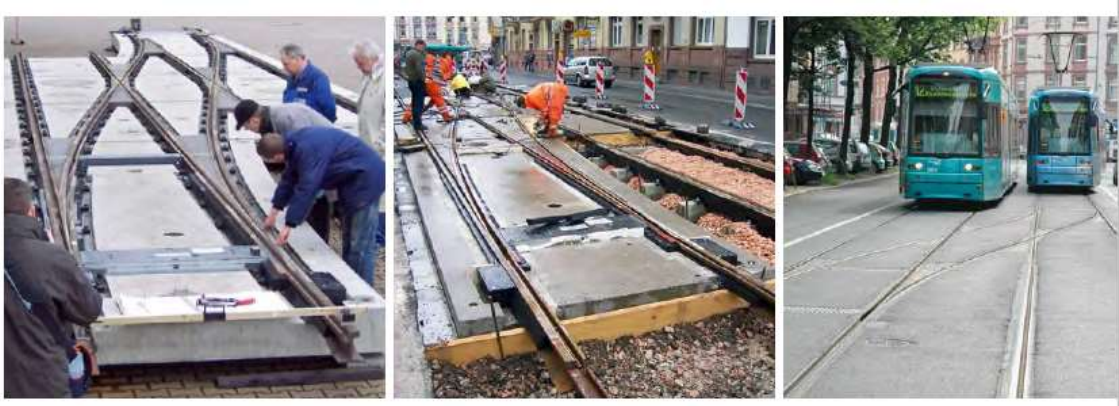
1. Installation and assembly of a turnout in a prefabricated slab – Frankfurt 2008 [4]
