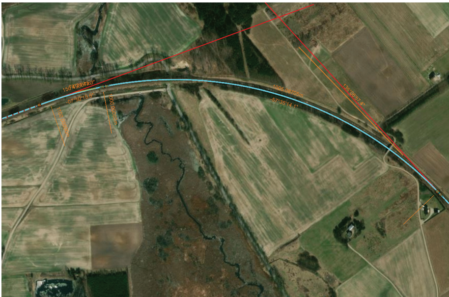
3. View of the layout of the reconstructed section
